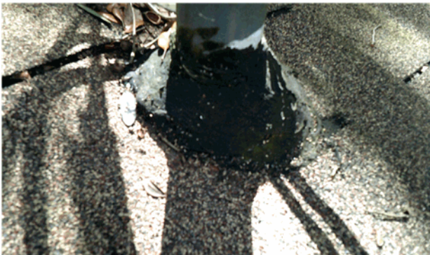
Electrical roof penetration
